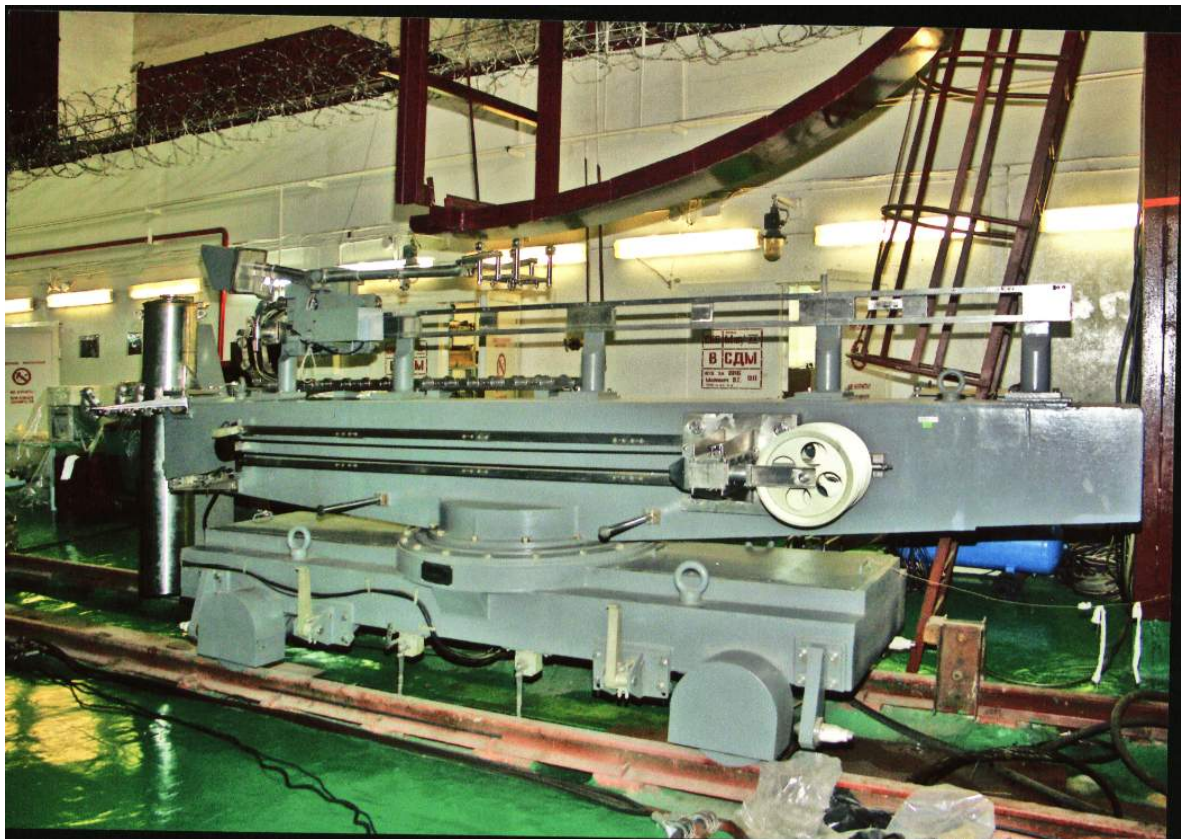
Fig. 3 SK-187 manipulator in SU NPP (stage 2)
